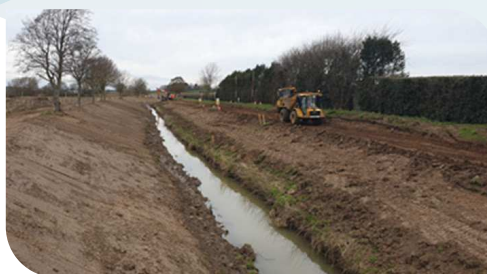
The Environment Agency's Stokesley Flood Defence Scheme in North Yorkshire. Augean managed 10,700 tonnes of dredgings at its treatment facility to process wet silts, dehydrating the dredgings with stabilising APCr to make suitable for disposal.
