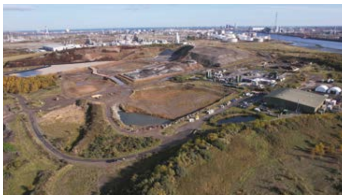
Aerial view of Augean's Port Clarence Site
