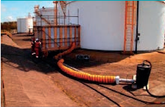
Ventilation Set-Up for Inert Tank Entry Clean
