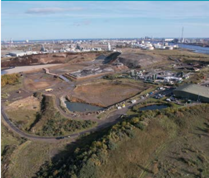
Augean's Port Clarence Treatment & Disposal Facility
