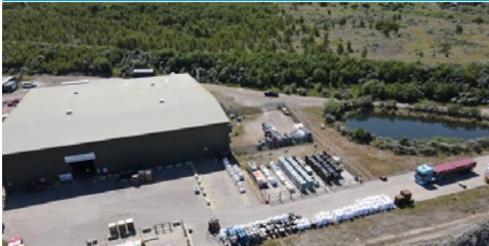
Aerial view of Augean's Waste Recovery Park with a consignment of combustible waste from Sellafield Ltd being delivered by Tyson H. BurrIDGE
