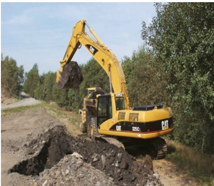
Plant extracting contaminated soil
